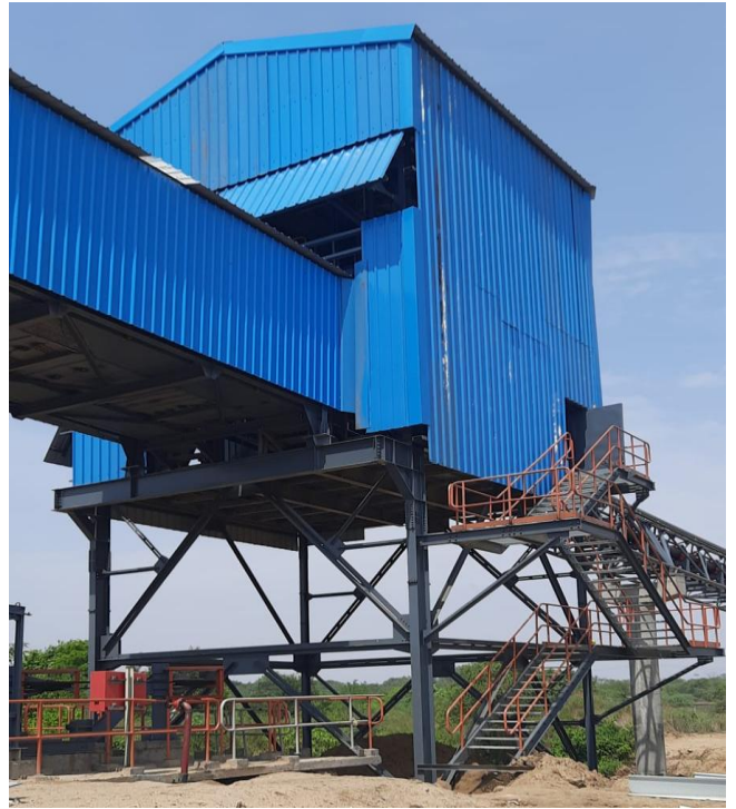
Cladding at DST-02
