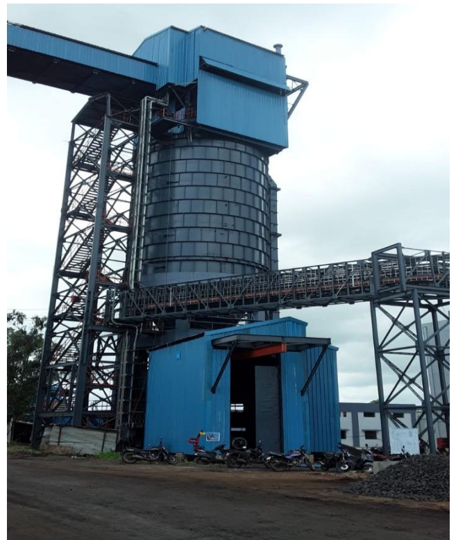
Cladding at Surge Hopper at Bhatadi
