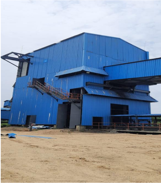
Cladding at Junction house – JH01
