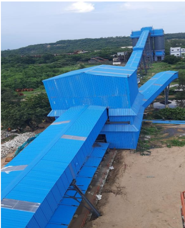
Cladding at PC tail end, BC-04, BC-02 & WLS
